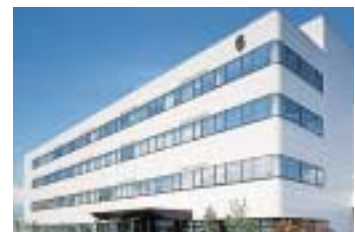
The new Process Technology Center in Nirasaki, Japan, is an advanced facility that supports the shift to 300mm equipment.
